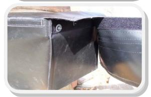
Head curtain can be easily replaced separately without disturbing the entire head member .
